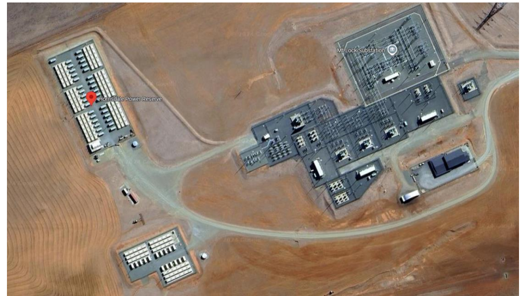
The main battery bank in the North West corner of Hornsdale Power Reserve in Australia measures 55m x 118m, equivalent to just 1.6 Acres. Developed parts of the site occupy under 8 acres. © Google Maps
