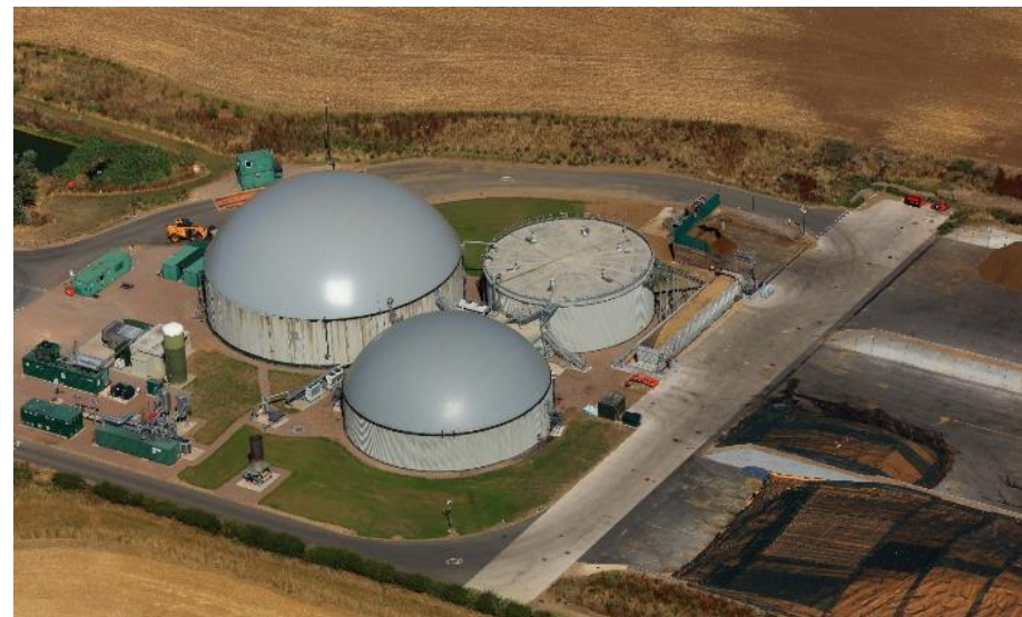
Typical anaerobic digestion facility. Biogas can be produced from waste and used to generate electricity. © Renewable Energy Association
