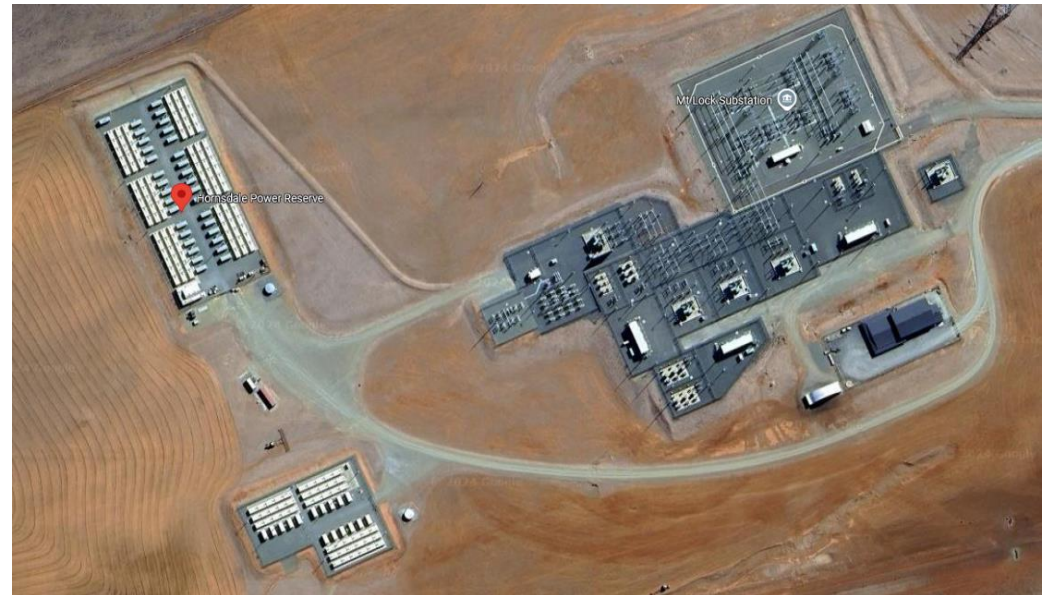
The main battery bank in the North West corner of Hornsdale Power Reserve in Australia measures 55m x 118m, equivalent to just 1.6 Acres. Developed parts of the site occupy under 8 acres. © Google Maps
